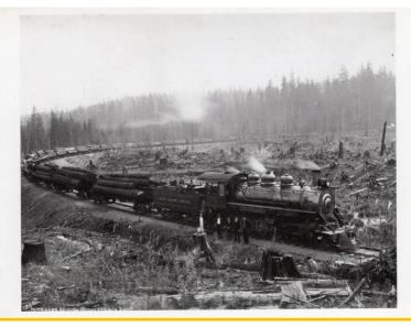
Pulling a large train of logs, this 2-8-2 steam locomotive is a Mikado built by the American company Baldwin Locomotive Works and owned by the Siler Logging Company in 1924.
